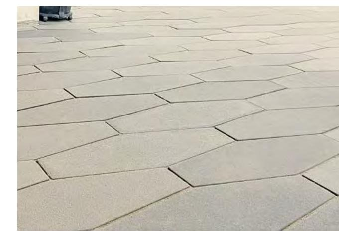
MATERIAL: PRECAST CONCRETE, MORTAR SET SIZE: 24" X 6" X 12" (DIAMOND) COLOR/FINISH: LIGHT BUFF/TAN, SANDBLAST
